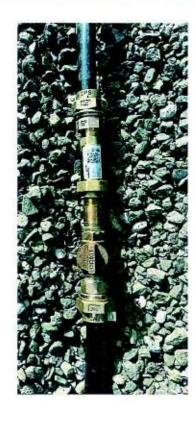
( %" female pac-joint to %" male threads, %" curb stop, 2" x %" brass nipple, in-line dual check valve, %" male threads to %" female pac-joint, will need 2 inserts for pipe)
