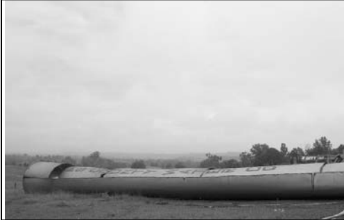
Locust Grove Tank Demolished !
